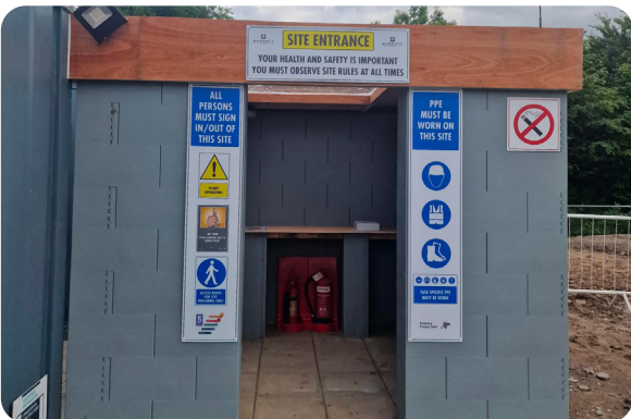
SITE HEALTH & SAFETY SHELTER
