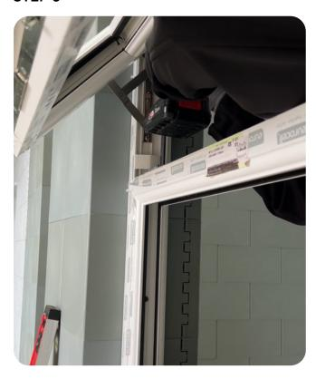
Screw in at the sides and checking it's level as you go.
