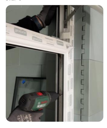
Using a countersink bit here just make sure that the screws don't stick out and disturb where you are going to place the glass panes in.
