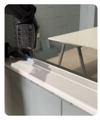
Once you receive your made to order window, make sure the sill fits in place. Then measure out and mark where the screws will go into the capping pieces.
