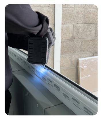
Begin to attach the frame to the sill on the bottom.
