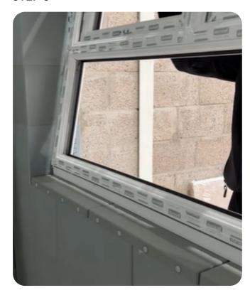
Push it into the opening and make sure it is level with the wall.
