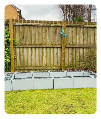
To lay the bottom layer, place two blocks side by side with their short sides touching at the left end of the footprint, then repeat the same at the right end. Next, position another four blocks in the middle (both sides) with their short sides touching, but place these inside the structure line so it sits slightly inset from the perimeter. Ensure all blocks are aligned, evenly spaced, and pushed tightly together to form a straight and secure base.
