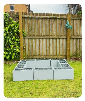
To lay the bottom layer, place two blocks side by side with their short sides touching at the left end of the footprint. Next, position three of blocks in the middle with their short sides touching, but place these three outside the structure line so it continues the square around the perimeter. Do the same on the other side. Ensure all blocks are aligned, evenly spaced, and pushed tightly together to form a straight and secure base.
