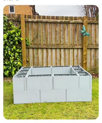
For the next layer, place the QUICKBLOCKs on top of the base in a brickwork pattern, ensuring that each block overlaps the joints of the layer below. Position the blocks so that the overhang is equal on both sides, keeping the structure balanced and aligned as you build upward.
