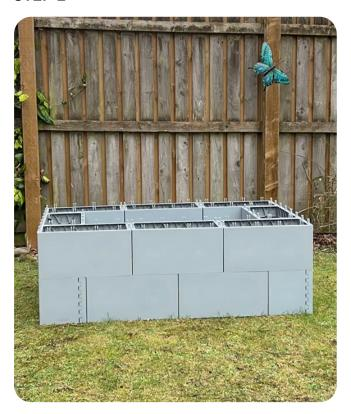
For the next layer, place the QUICKBLOCKs on top of the base in a brickwork pattern, ensuring that each block overlaps the joints of the layer below. Position the blocks so that the overhang is equal on both sides, keeping the structure balanced and aligned as you build upward.
